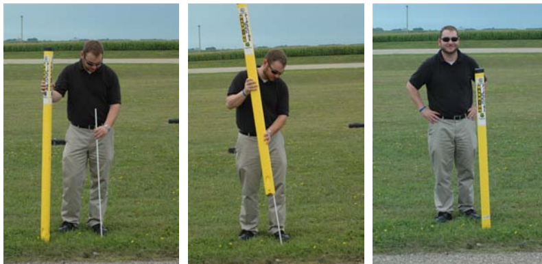
1. Insert Flex-PLUS rod in hole/anchor
