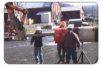
Western Plant & Pipeline Products Inc. has picked up a new product called The Safeway Pig Loader. The Safeway Pig Loader is a much safer method of hand launching pigs compared to the traditional push rod and backhoe.
